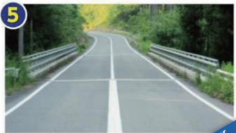
Material transportation road
