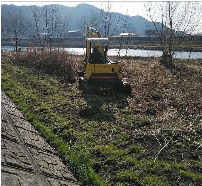
[高水敷整正（再繁茂対策）] 狩野川右岸3.0 km
