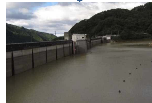
②洪水調節後(10/13 8:00頃) EL.446.72m
