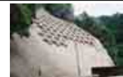
道路法面防災対策
