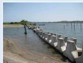
変形護岸の締め切り(下坂手)
