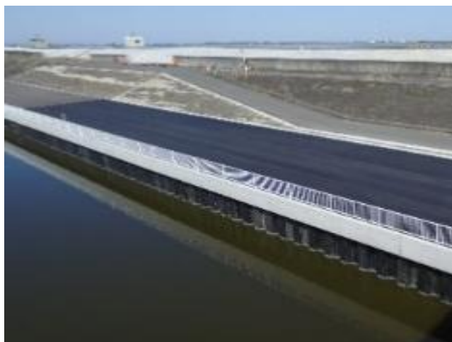
矢板護岸の補修
