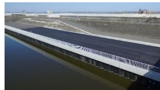
矢板護岸の補修
