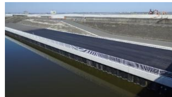
矢板護岸の補修
