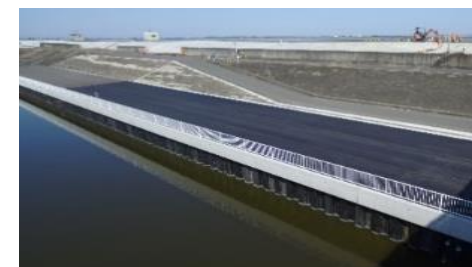
矢板護岸の補修
