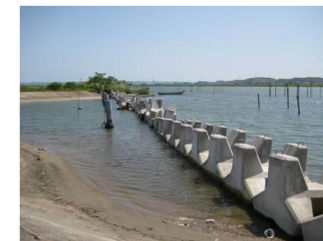
変形護岸の締め切り(下坂手)
