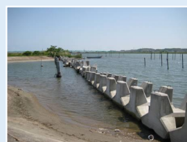
変形護岸の締め切り(下坂手)
