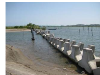
変形護岸の締め切り(下坂手)
