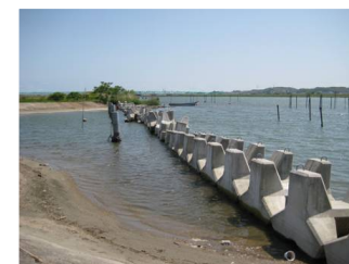
変形護岸の締め切り(下坂手)
