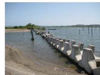
変形護岸の締め切り(下坂手)
