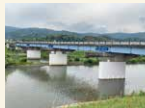
橋梁の耐震補強
