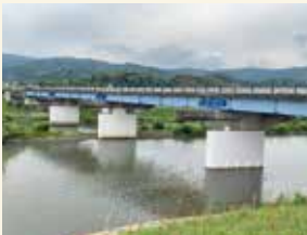
橋梁の耐震補強
