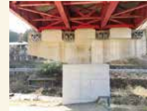
橋梁の耐震補強
