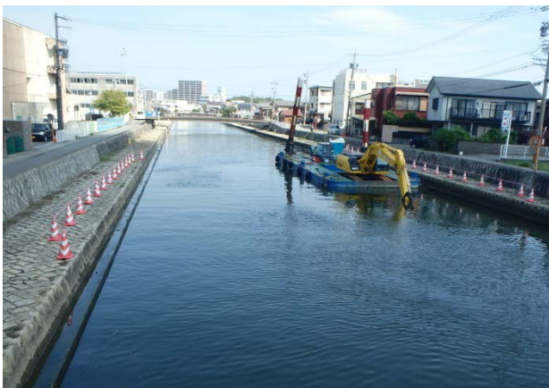
No. 2 勢田川河道掘削
