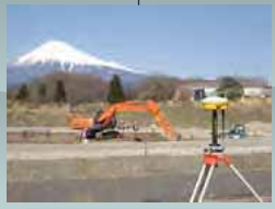
ICT施工 (MG)
