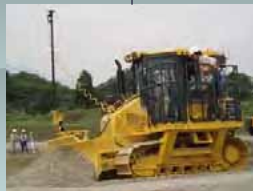
ICT施工 (MC)
