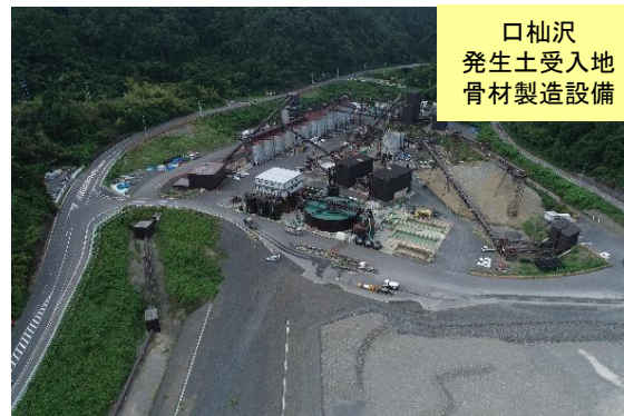
施工内容：骨材製造工 (Construction content: aggregate manufacturing work)
