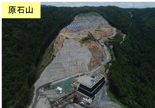
施工内容：原石山の表土掘削、原石採取 (Construction content: surface soil excavation and original rock collection)
