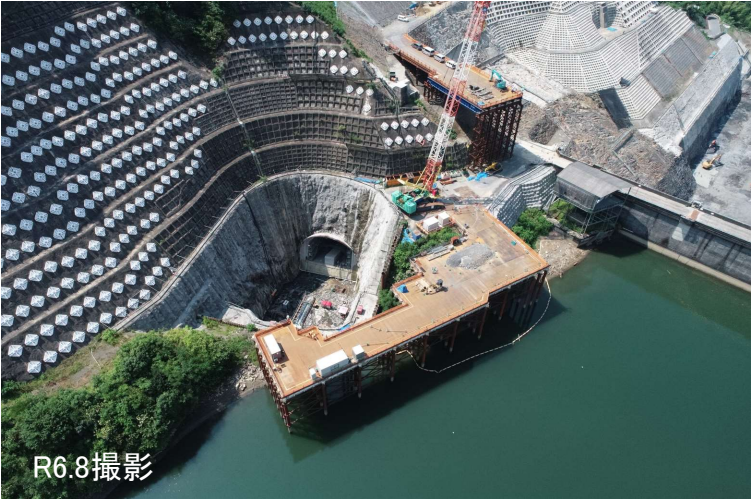
転流工呑口部現況 (Current status of diversion work inlet section)
