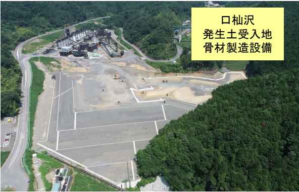
施工内容：骨材製造工 (Construction content: Aggregate manufacturing work)
