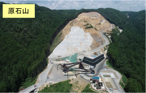
施工内容：原石山の表土掘削、原石採取 (Construction content: Surface soil excavation and original rock collection)
