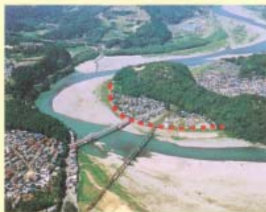
②北鹿島築堤
