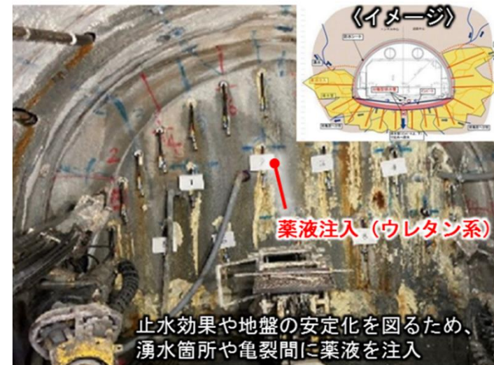
＜注入工（地山改良工）＞
