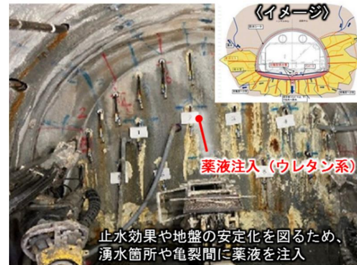
＜注入工（地山改良工）＞
