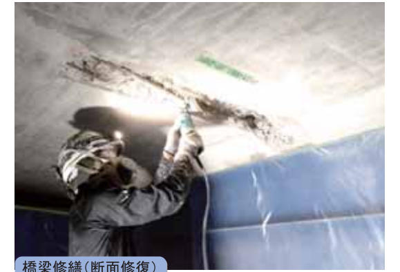
橋梁修繕(断面修復)
