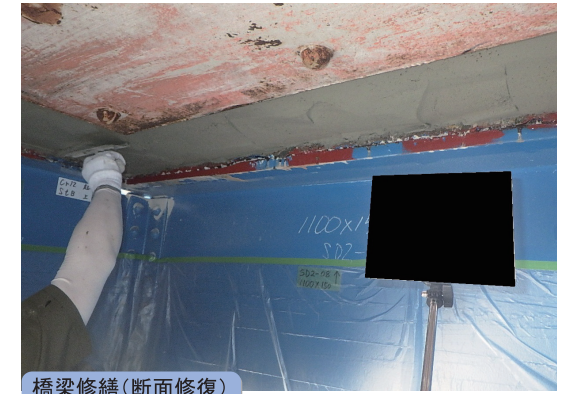
橋梁修繕(断面修復)
