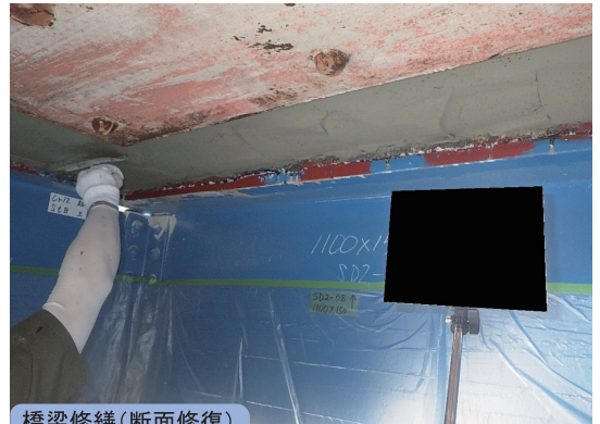
橋梁修繕(断面修復)
