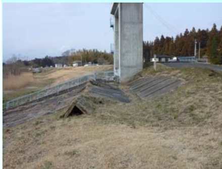
護岸の破損
