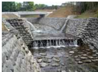
Okubosawa stream preservation works
