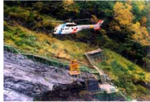
Concrete placement by helicopter
