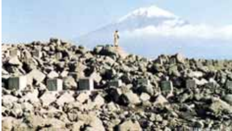
Sedimentation condition of debris flow at the 9th groundsill of the Osawa sand pocket (November 28, 1991)
